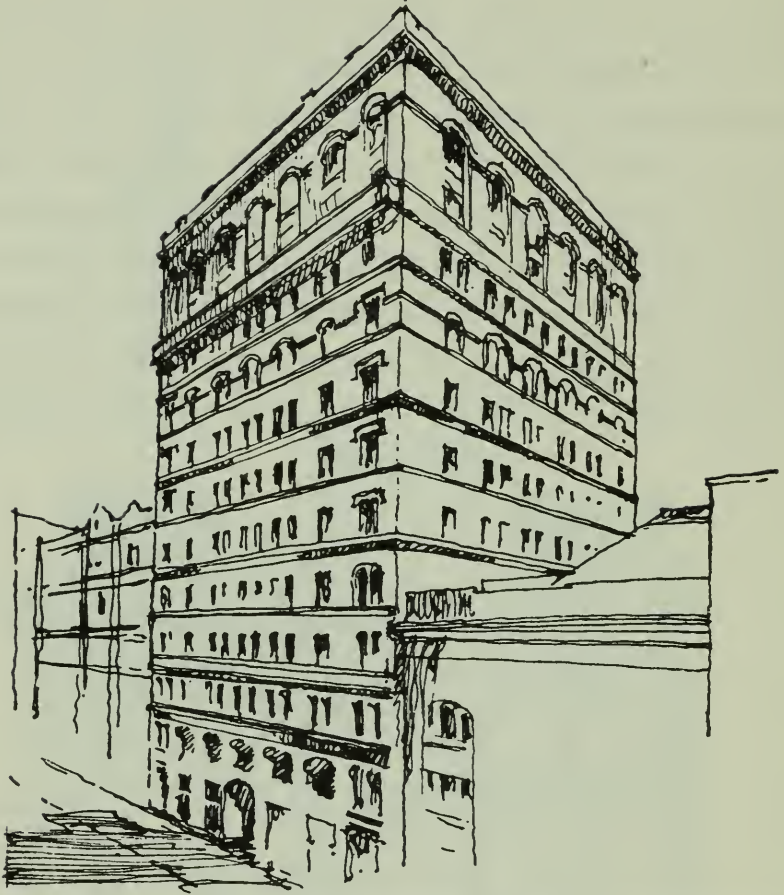
FIG. 39.—A New York office building. Indecision through continual stressing of horizontals in a vertical mass.
